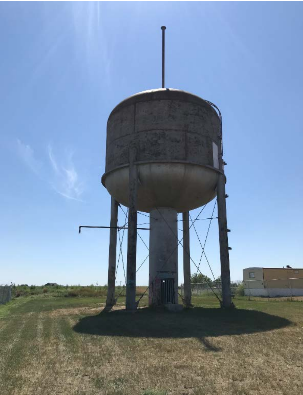
Image 2. 317 – 1 st Avenue, Tower (2021)
