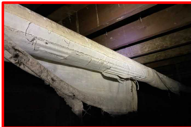
A2- Pipe Insulation/Basement
