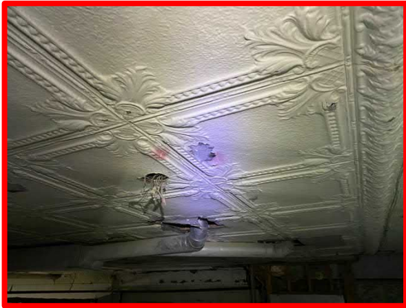
L1- White Paint / Bathroom 2 nd Floor
