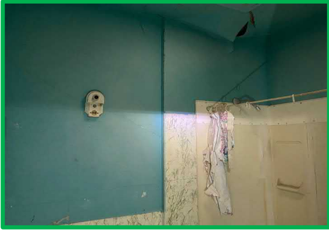
A7- Wall Plaster/ Bathroom 2 nd Floor
