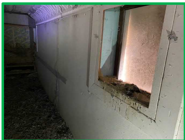
Sample A5- Wall Plaster/ Back Exterior Wall
