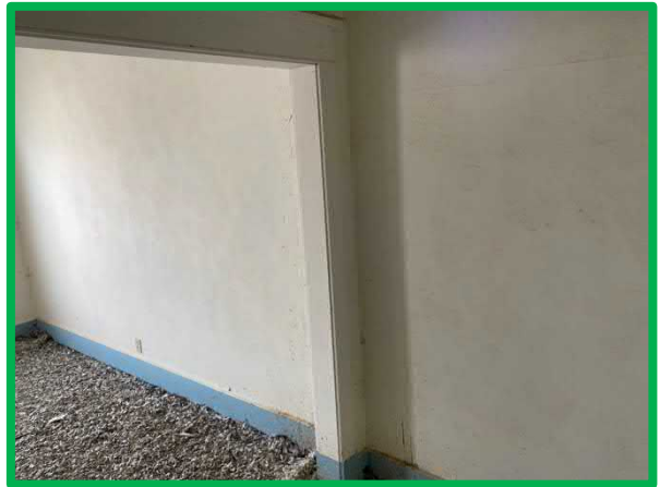
A8- Wall plaster 2 nd Floor; Front Exterior Wall
