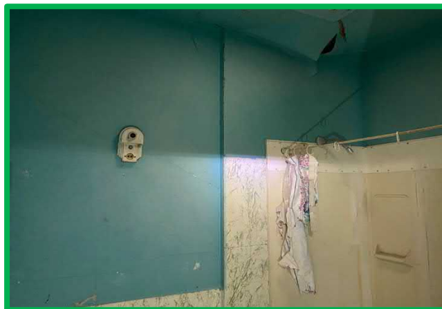
A7- Wall Plaster/ Bathroom 2 nd Floor
