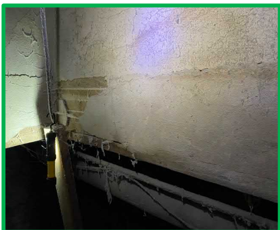
A3- Wall Plaster/ Basement
