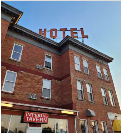
The Imperial Hunter Hotel in the Town of Bassano, which operates under Class A (Minors Prohibited) and Class D (General Off Sales, Hotel) licences.
